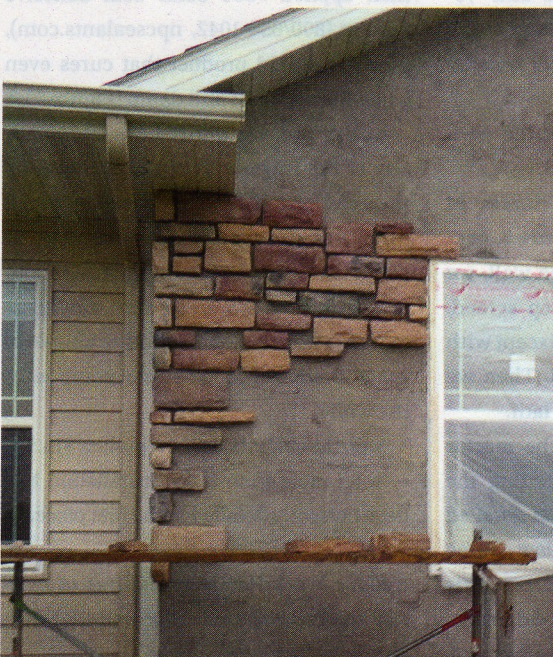
Figure 6. Like stucco, manufactured-stone veneer is applied over a base coat of mortar (left). The cap flashing (above) is sized to match the thickness of the stone veneer, to ensure that water is diverted to the surface.
