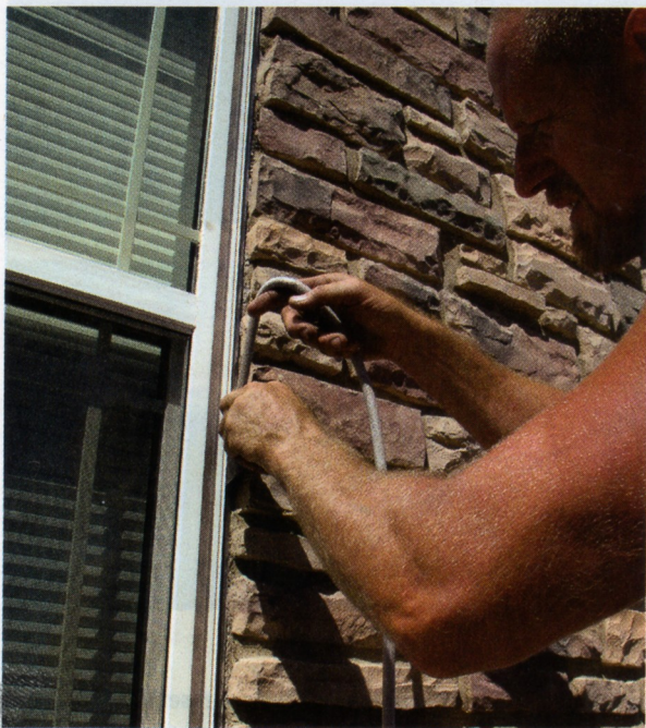
Figure 7. Backer rod inserted between the metal J-mold and the window frame (above) prevents the sealant used to fill the gap (above right) from adhering to the back of the joint, allowing it to remain flexible without pulling away from the sides. At right, the finished wall.
