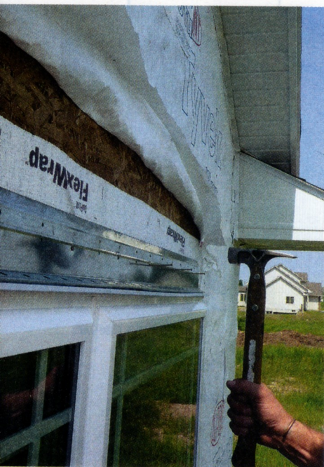
Figure 4. A metal weep screed above the window allows water to drain out from behind the cladding and mortar base coat (left). Metal J-mold is applied underneath the window (above left) and at the jambs (above right); flexible sealant is used to fill the joints between the J-mold and the window.
